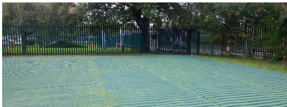
The freshly-laid ground mesh covering the front lawn.
